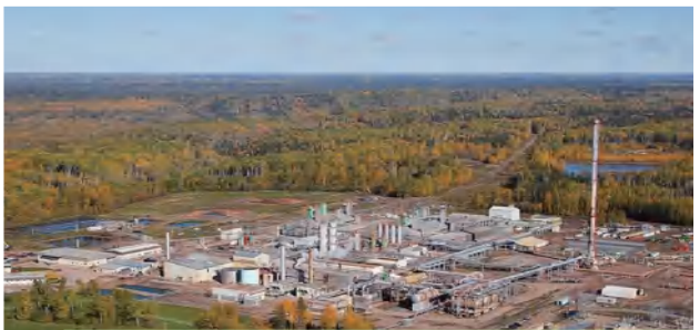
Canada 1000m 3 Hydrogen Project ZHSZCB-5800/35kV Hydrogen Production Dry Type Rectifier Transformer
