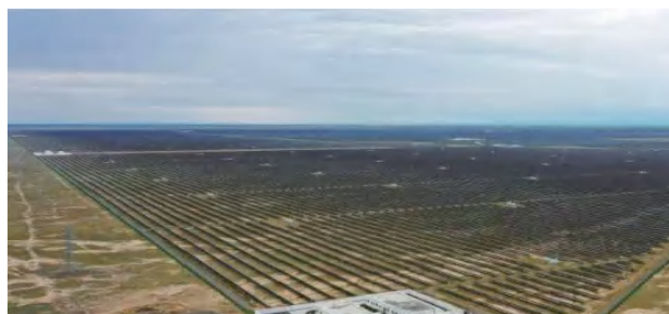
Xinjiang Mulei 125MW Energy Storage Project SC(B)-2800/37kV Cast Resin Dry Type Transformer
