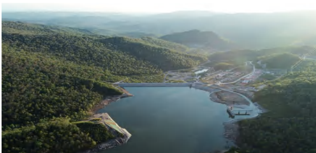
Changjiu new materials Pumped-storage Project KSG-1000/10kV Mining Dry Type Transformer
