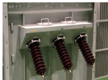
hand hole structure
